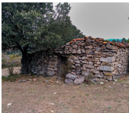
Shelter in the Noguerón of Beamud / JLS
